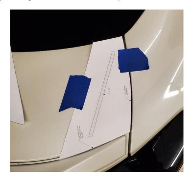
2.8. Begin cutting the top skin out by following the guidelines on the template. You can use a 1/4" drill bit on both ends, and a cut-off wheel to cut out the slot. This should give the slot a nice clean radius. NOTE: Be sure to use a vacuum to clean out all the metal chips before moving on.
