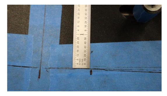
**3.9.** Confirm that the marks line up with the mounting tabs correctly before drilling.
