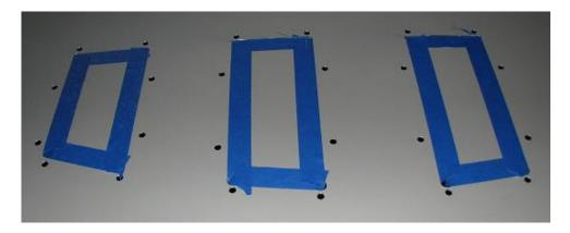
2.17. Using the cut-off wheel and the straight grinder, carefully follow the edge of the blue tape to help you keep the cut straight. There is no rush. This is the hardest part of the install, so take your time and don't get hasty with cutting through the aluminum. Note: It is much wiser to place the blue tape on the outside, not the inside as shown.
